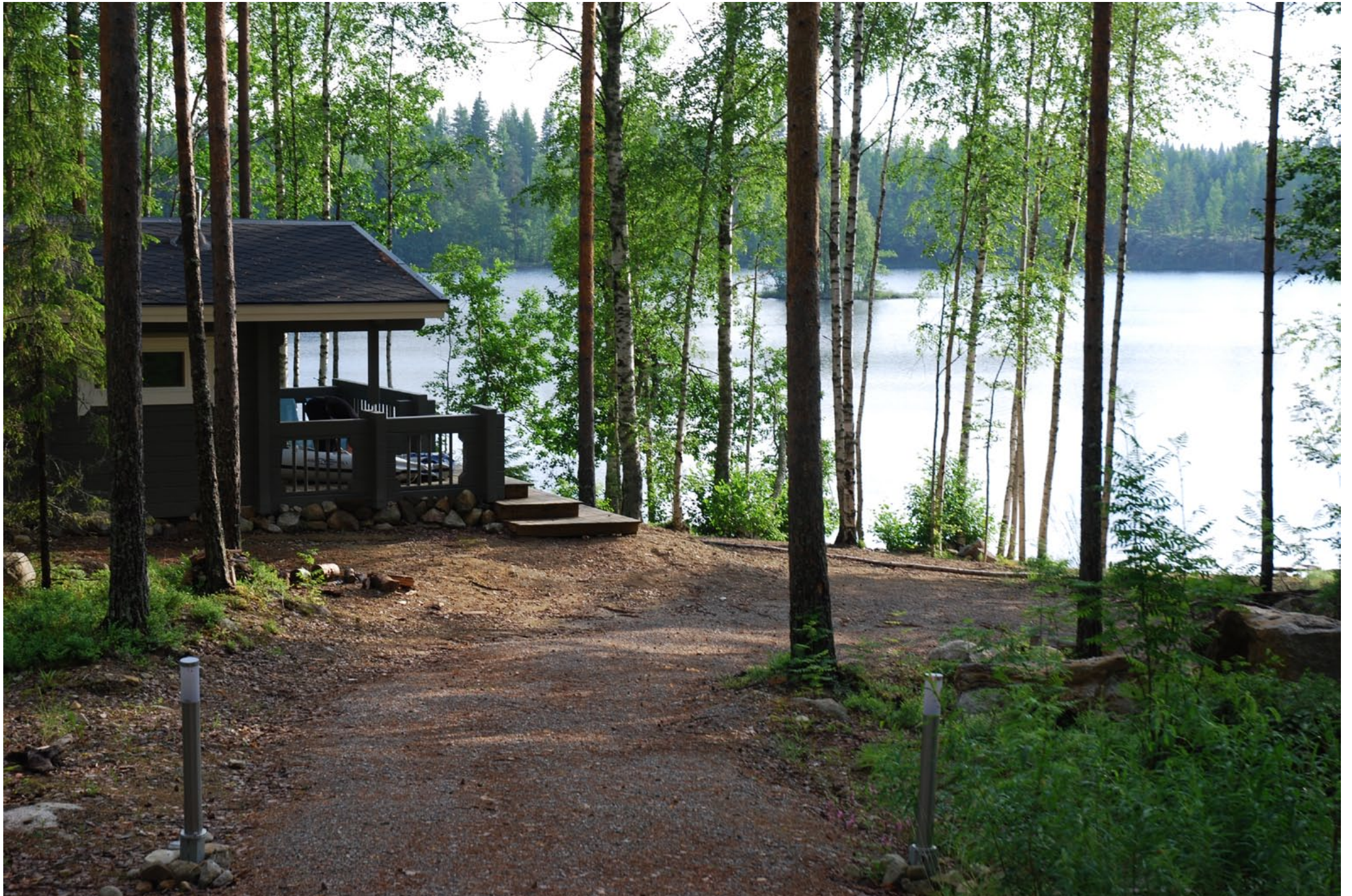
GUEST HOUSE: a birch bath with a guest house function. Area 25 m 2 , 2 entrances.
